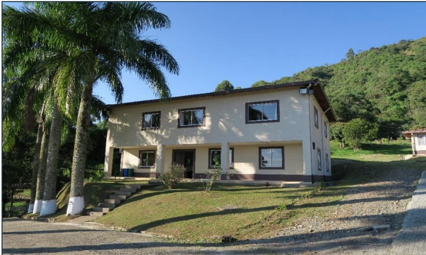
La Mina Office
