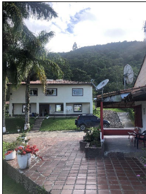
Figure 12-3 Geology office and accommodation house
