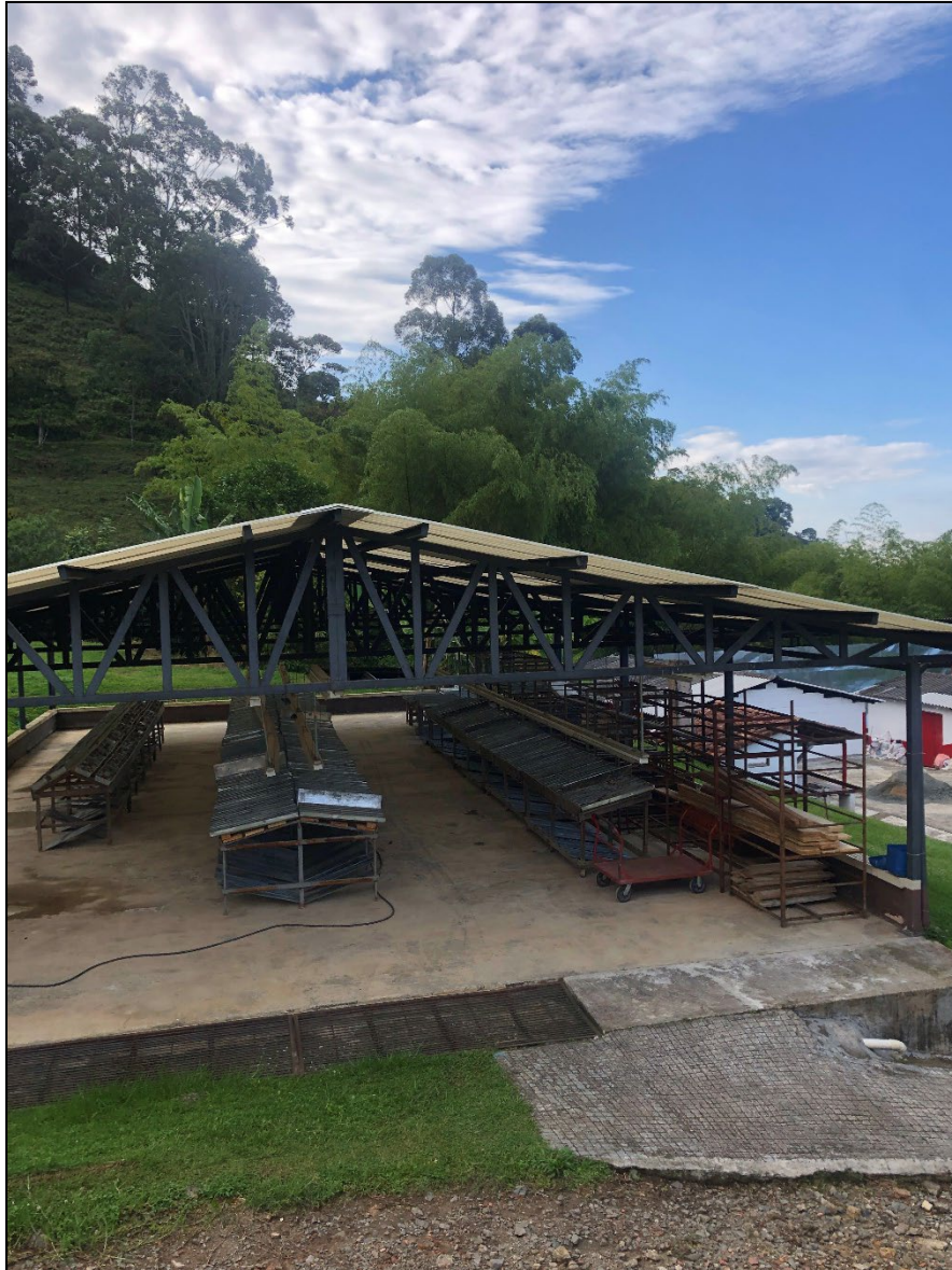
Figure 12-7 Core shed for core logging and sampling
