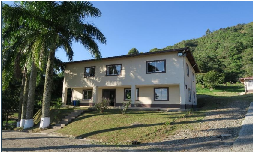
La Mina Office
