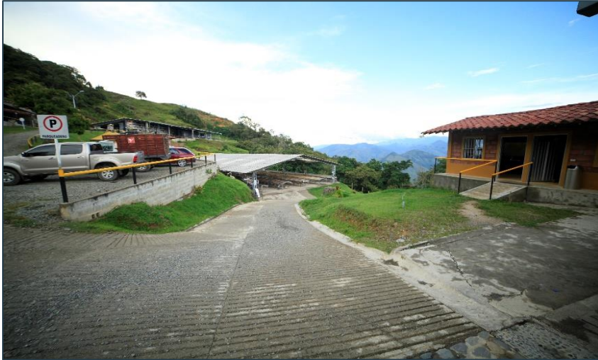
Titiribi Office and Core Facility
